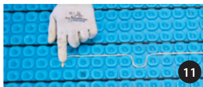
11 Install the floor sensor between 2 cable runs.
