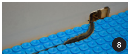
8 Start the installation of TRUE COMFORT Cable by cutting the membrane to insert the mechanical joint and part of the cold lead.
