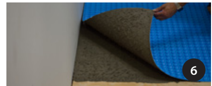
6 Check the thinset mortar transfer to the membrane. In case of partial coverage, increase the amount of adhesive or its fluidity.
