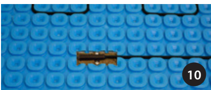
10 Finish the cable's installation by cutting the membrane and inserting the end of the cable.
