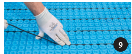
9 Insert the cable according to the installation guide, making sure not to exceed a maximum output of 15W/ft 2 .
